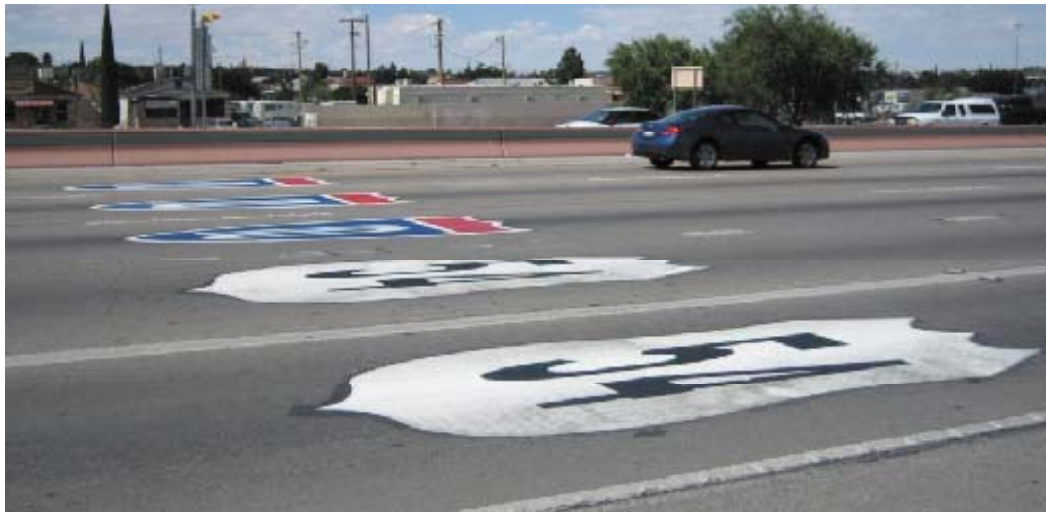
Figure 1. Example of In-Lane Pavement Marking Shields
